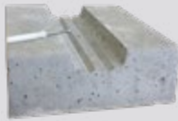
concrete footing + hammer plug
