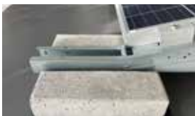
Concrete footing + anchor
